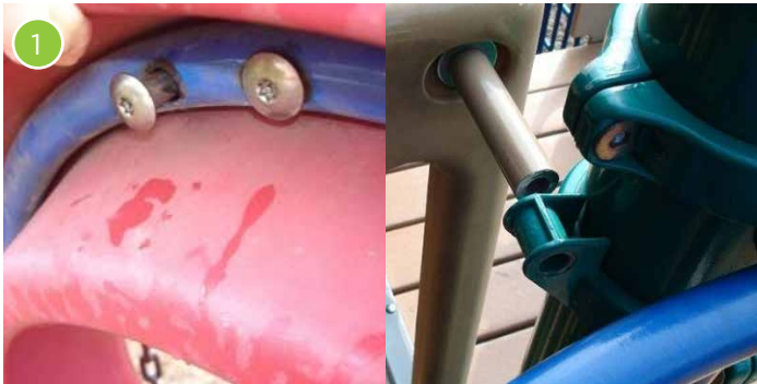
This bolt is loose and should be tightened or replaced.
